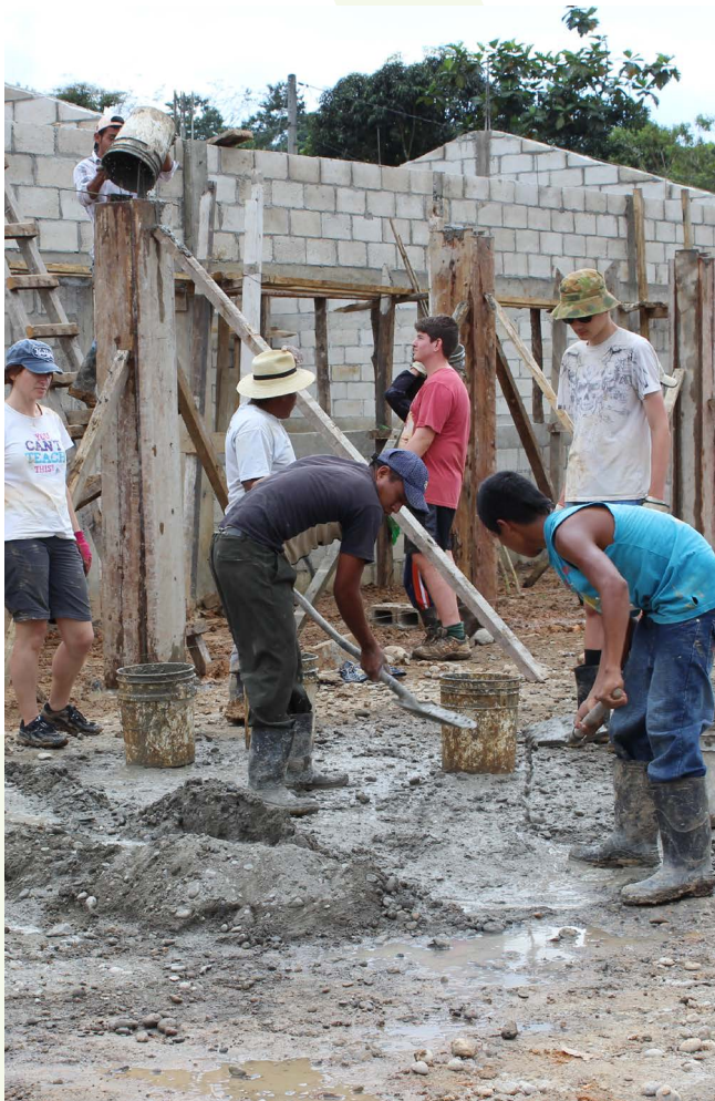
The construction site
